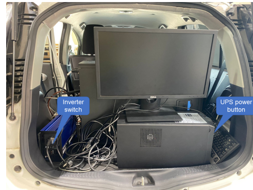
Figure A.2: Inverter and UPS on ATLAS-CAR2.
